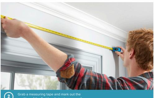
position of the first bracket using a pencil.
