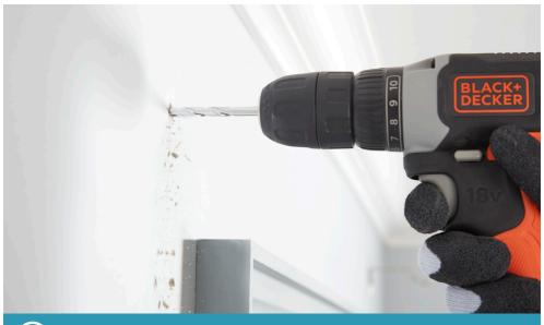
(7) Once more, check for any cables, then drill the holes and fit the bracket as before
