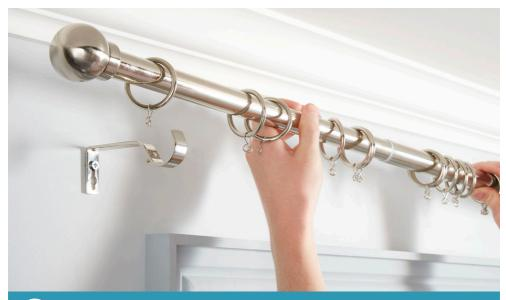
Finally, add the curtain rings and fix the poles to the brackets at each end.
