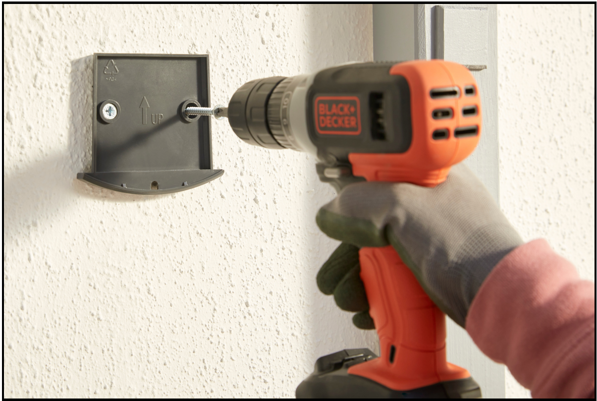
7) Fix the mounting plate to the wall.
