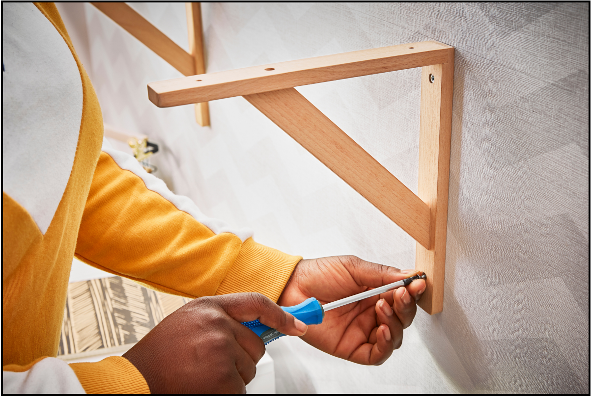
7) Screw both of the brackets into place.
