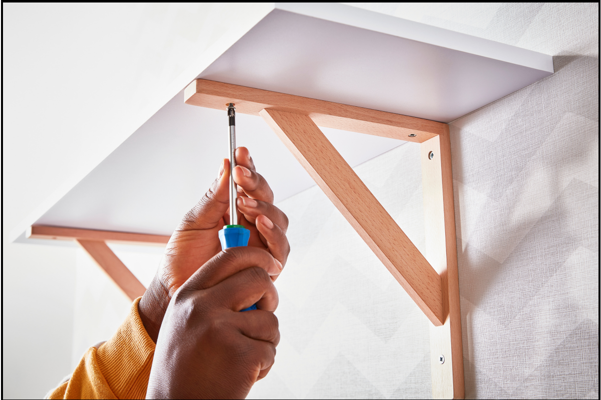
8) Finally, fit the shelf, securing it to the brackets on the underside with a small screw. And that's it – job done!
